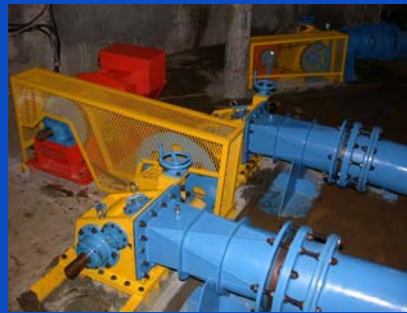
BSB, Cisarua, Jabar X-flow T-14, ELC-25 kW-Mini-Grid 2004
