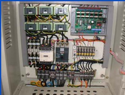
Electronics Load Controller PLTMH Dadapan, Sumatera Selatan ELC-MC1 HeksaHydro- 30 kW
