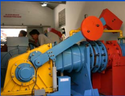
X-flow Turbine T-14 D300 head: 3 – 100 meter power: 10 – 150 kW
