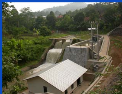
Melong, Subang, Jabar X-flow T-14 D500, ELC-100 kW-Grid PLN 2005
