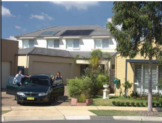
Photo: BP Solar
