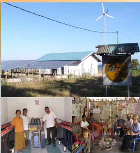
The E7 PV-Wind-Diesel (21.8 kWp-10 kW-20kVA) Hybrid System in Oeledo Village (Rote Island), May 2005.
