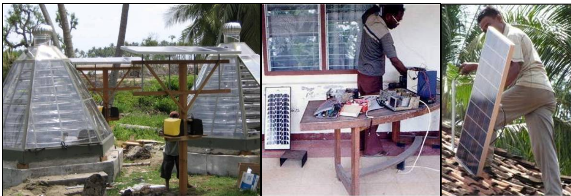
Fig. 3: (1) Fish solar dryer in Aceh using a combination of wind-sunlight and biomass sources (Photos courtesy of Azet Surya Lestari Co). (2). PVES used in the December 1992 tsunami in Maumere, Flores (NTT Province), deployed to power telecommunication during the emergency handling following the disaster (photo courtesy of Claus Dauselt). (3). The installation of a SHS in Lampung creating jobs for the local people (Photo: M Retnanestri 2005).
